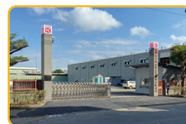
Zhongli Ziqiang Plant
